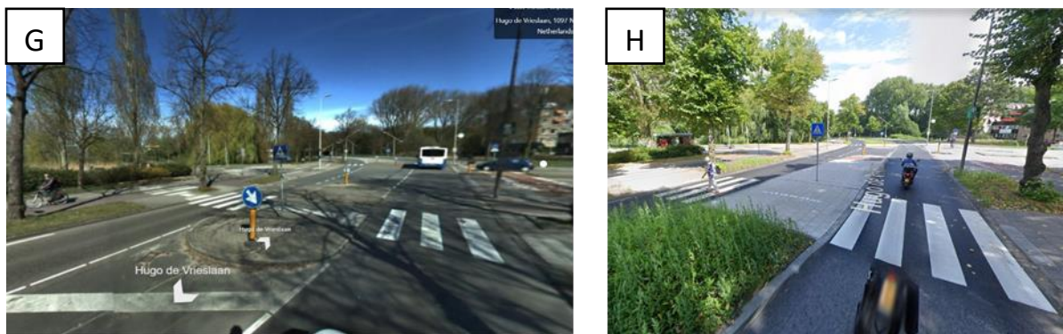
Fig. 12 : Transformations of the median strip West of the intersection with added raised curbs and added greenery of 80 m 2
