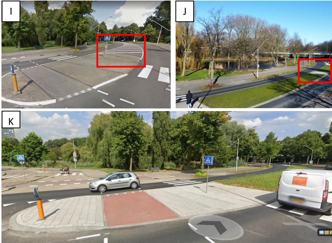
Fig. 13 : Median strip East of the intersection with added raised curbs and 300 m 2 of vegetation.
