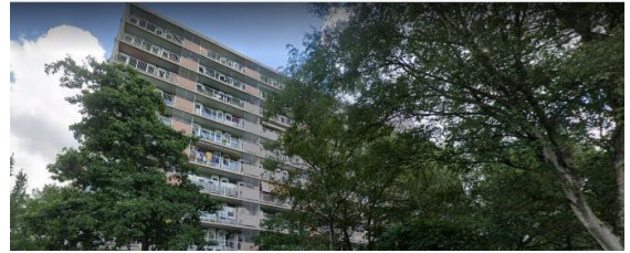
(b) West facade
