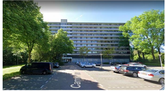
(c) East facade
