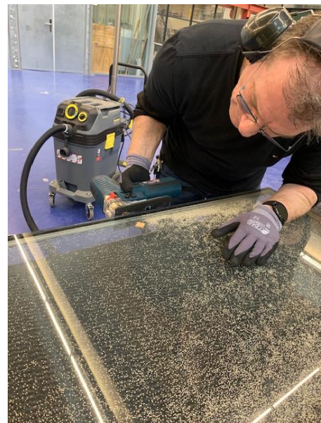
(d) Release of moisture-resistant granules between panes
