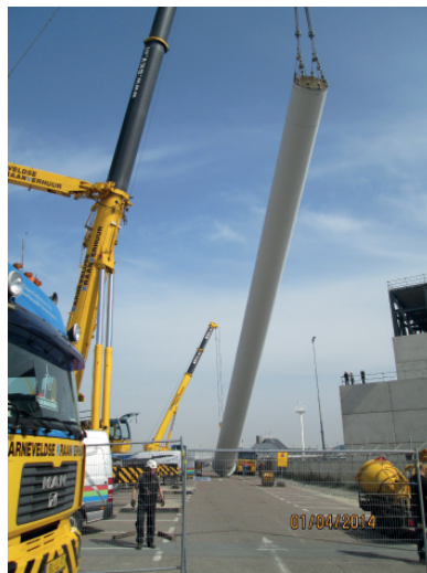
(c) Dismantling of the tower.
