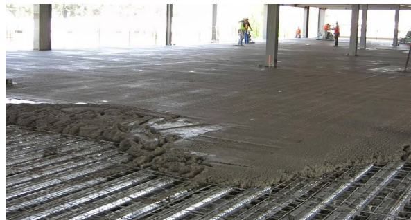
Figure 2.5: Composite steel deck floor [29]
