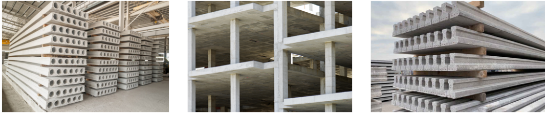
Figure 2.4: Concrete hollow floor, flat slab, T-beams [26, 27, 28]
