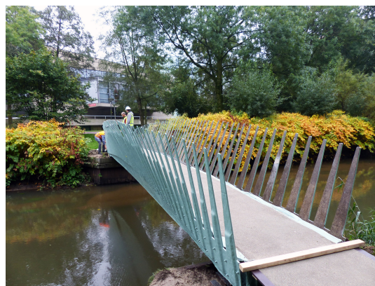
Figure 3.6: BFRP bridge at University Eindhoven
