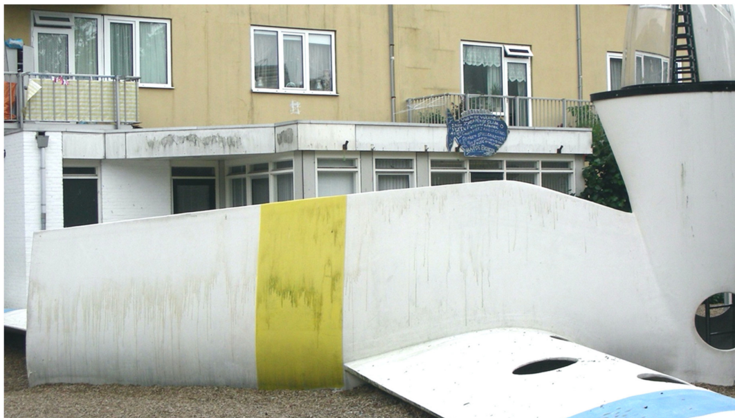
Figure 14. Leaching on the surface facing north-west of the blade standing on the long side (Photo by Piero Medici, 2011).
