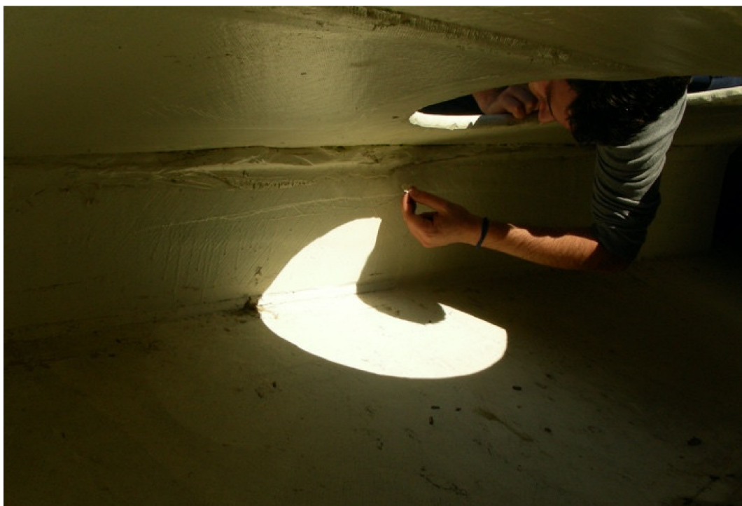
Figure 4. Interior of a rotor blade where finishes are cut and brittle as a consequence of the use by children. The interior of the blade is accessible; some parts are more than a metre high, where a young child can stand and walk. (Photo by Piero Medici, 2011).
