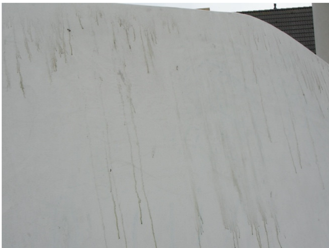
Figure 15. Drops leaching along the north-west surface of the blade standing on the long side (Photo by Piero Medici, 2011).
