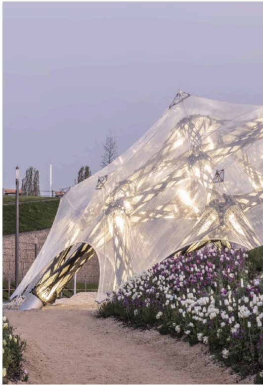
fig.06-23: buga pavilion, membrane
