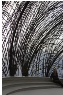
fig.06-06: gridshell FRP structure
