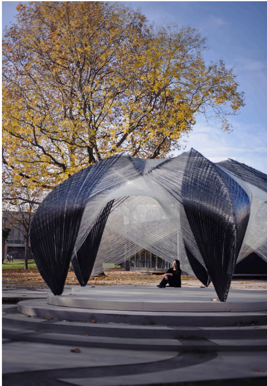
fig.06-08: research pavilion 2012 spanning 8 meters and 4mm shell thickness
