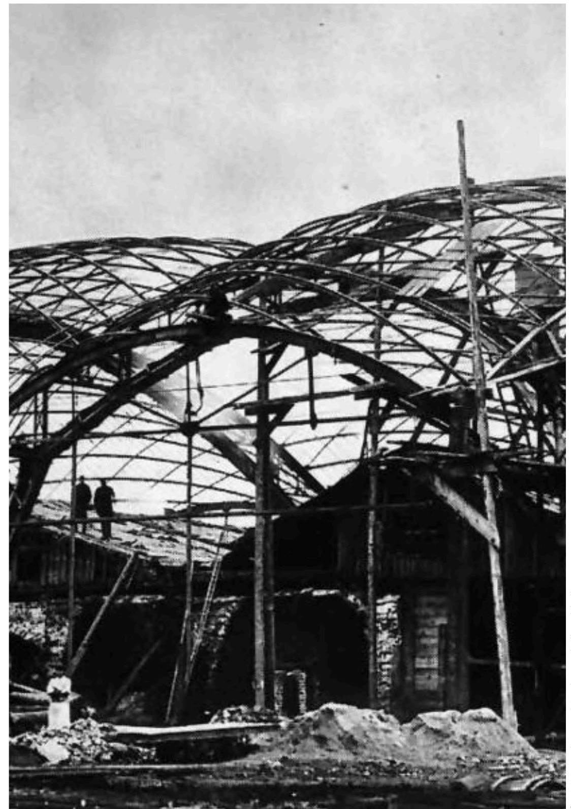
fig.06-07: vyksa steel Production hall gridshell structure
