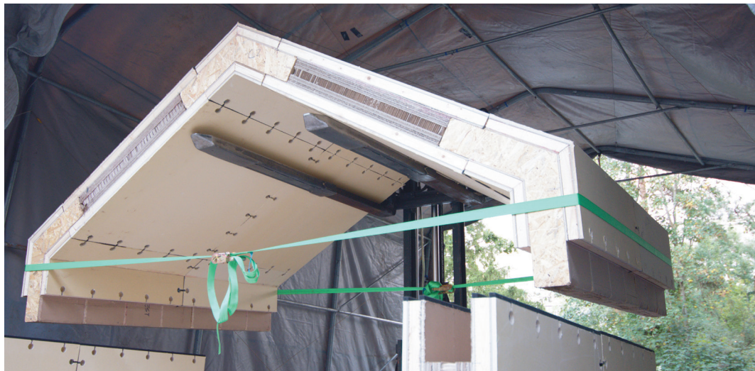
FIG. 10 Lifting the roof onto the construction
