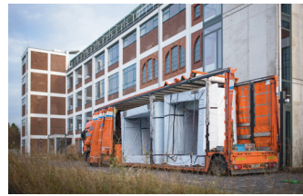
FIG. 13 transport of modules
