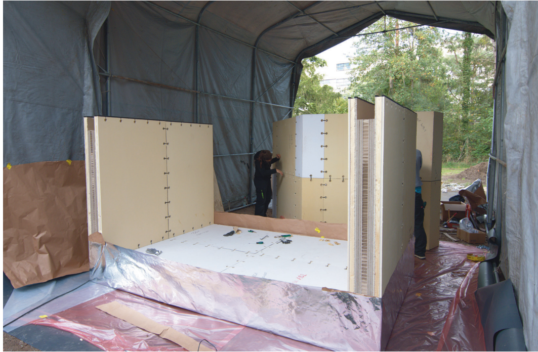
FIG. 9 Floor and wall modules. Assembly of the roof in the background
