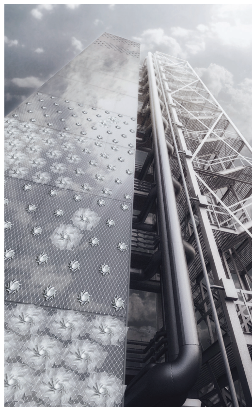
FIG. 12 Visualisation of the demonstrator high-rise building with adaptive membrane façades. Copyright by ILEK
