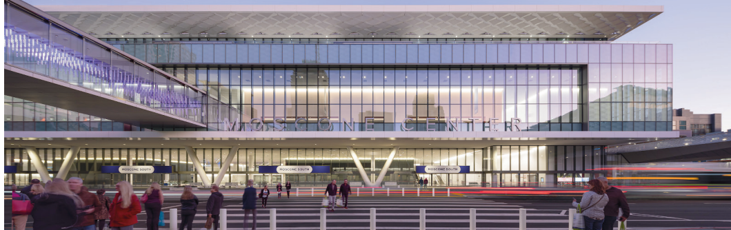
FIG. 1 Splash Page – Contextual introduction: overview image of building featuring the façade system(s), with project general facts/description/timeline
