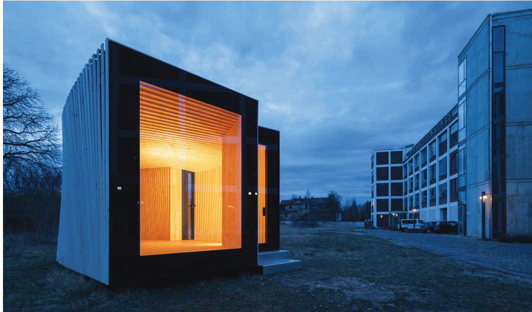
FIG. 15 Completed IBA: Timber Prototype House Demonstrator
