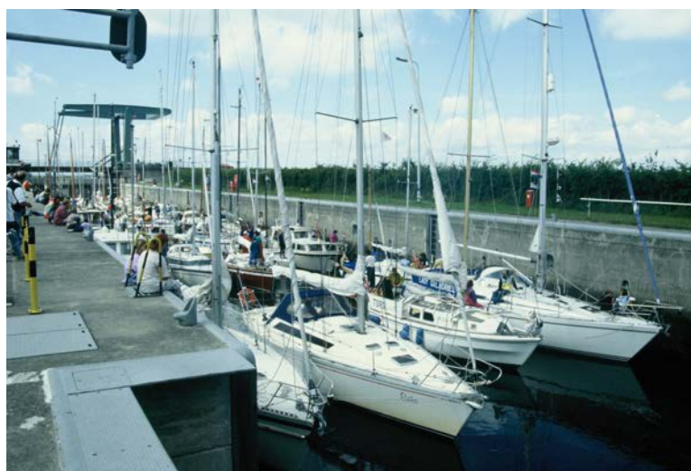
Figure 2.10: Locks are not only used by cargo ships (image by https://beeldbank.rws.nl , Rijkswaterstaat).
