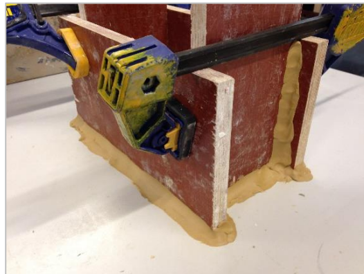
Step 6: Apply formwork and make sure all edges are made watertight by adding clay. Apply some Vaseline inside the mould for better demoulding.
