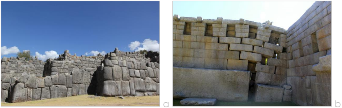
Figure 24: Inca megalithic interlocking stone walls (a), boundary induced failure (b). Reprinted from (Cervera, 2016).
