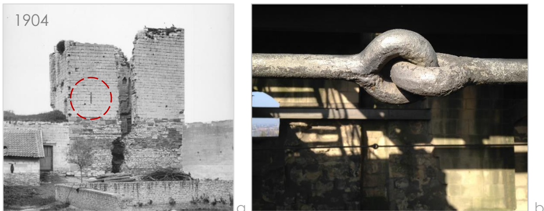
Figure 53: a) 1904 picture featuring a single intervention (see red circle); B) picture of measured tie rod. Adapted from: a) (Anonymous, Ruine Lichtenberg, 1904); b) photograph by author.
