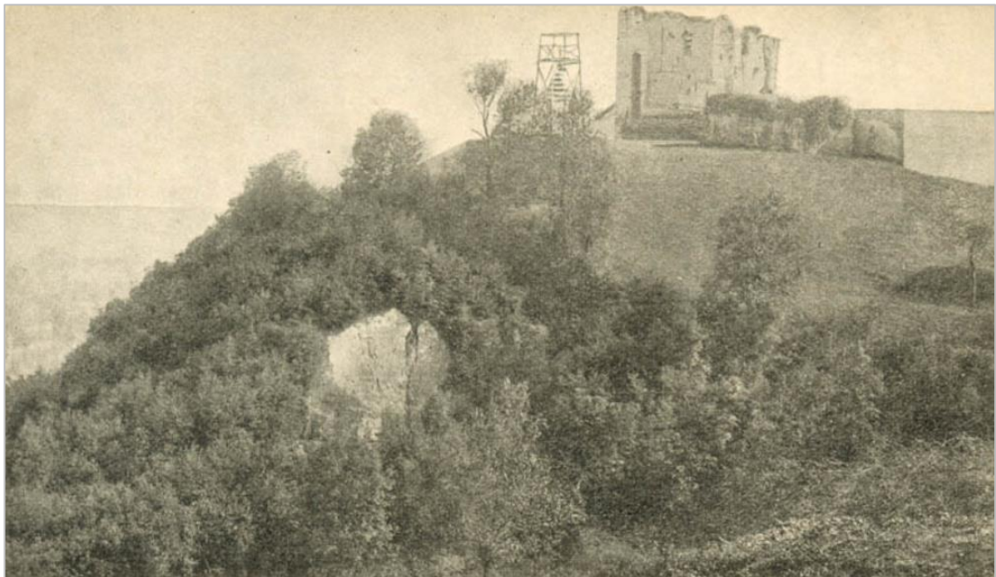
Figure 47: Photograph from 1900, depicting the ruin and its surroundings. Reprinted from (GAM, 1900).
