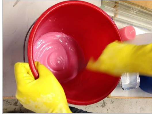
Step 8: Mix the two components thoroughly into an even mixture.
