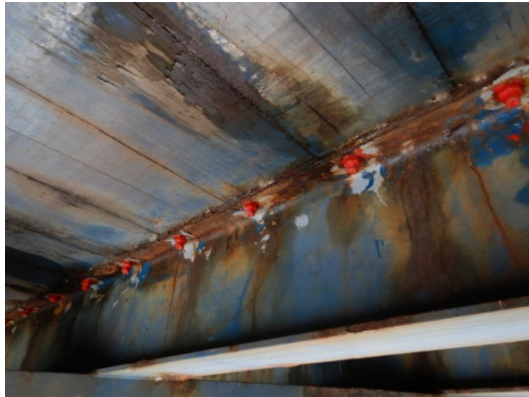
Figure 3.2: Timber deck to secondary girder connections
