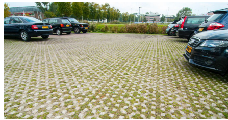
(c) Example of permeable pavement on a parking lot (Michon, 2018).
