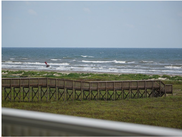
Figure N.3: Front side of a Dune walkover on Galveston Island West End at Kahala Beach.
