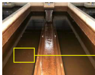
(b) Full-scale RSF during ETSW 5 m/h up-flow (c) Full-scale RSF during ETSW bed, spouting channels
