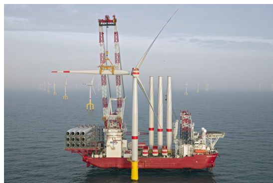
Figure 2.2: Wind turbine blade installation by jack-up Seajacks Scylla.
