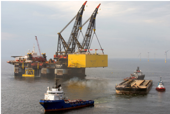
Figure 1.1: Thialf during installation of the Dolwin Alpha converter station.
