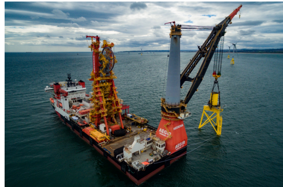
Figure 1.2: Aegir installing an offshore wind turbine jacket at Aberdeen.
