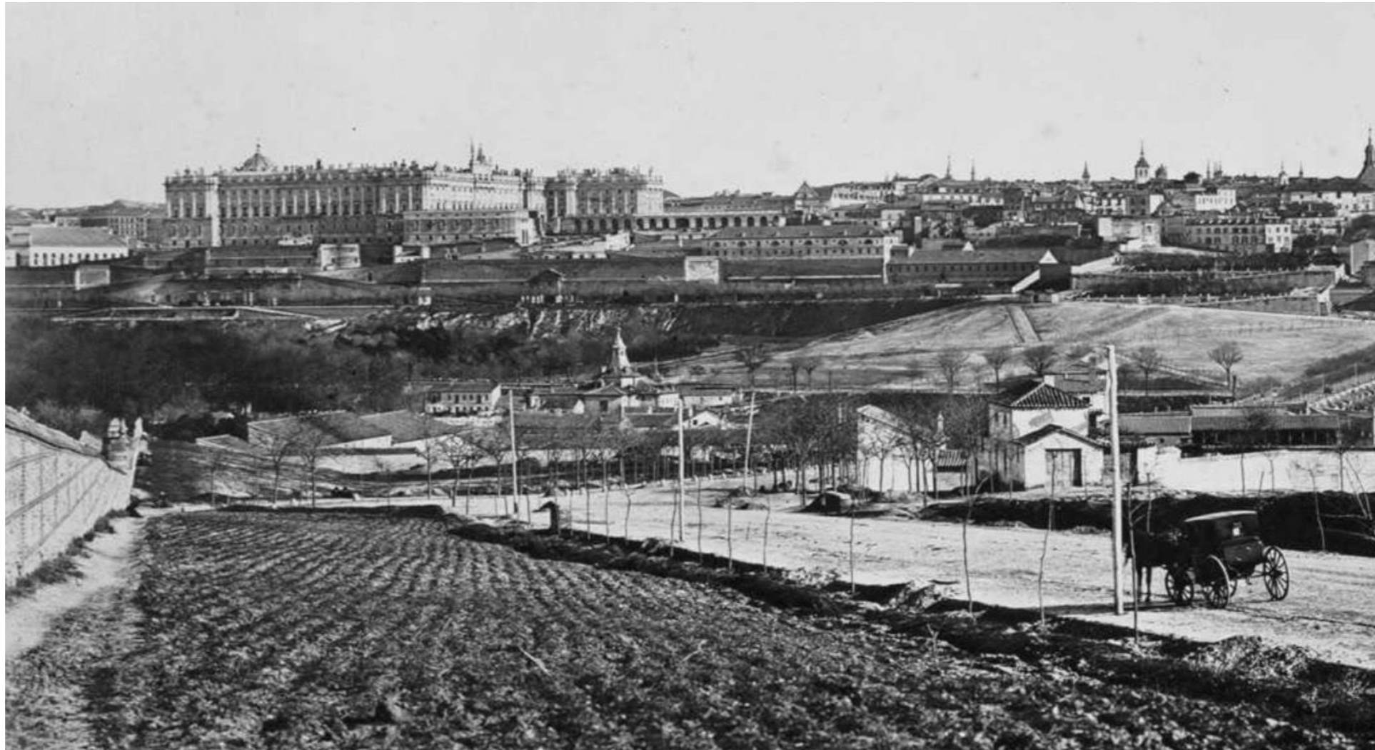
Views of the west bank of the Manzanares River around 1900
