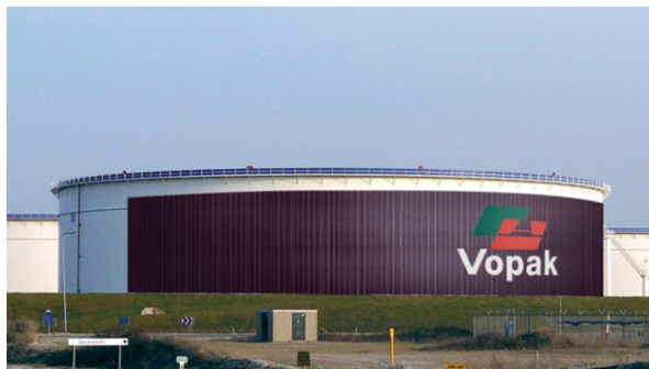
Figure 1.4: An artist render of Hyet thin-film silicon modules on a Vopak terminal [17]
