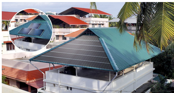
Figure 1.5: An artist render of HYET thin-film silicon modules compared to c-Si modules on a rooftop [19]
