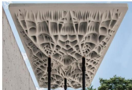
Figure 3.11 Optimised concrete slab prototype A. From (Jipa, Bernhard, Meibodi, & Dillenburger, 2016).
