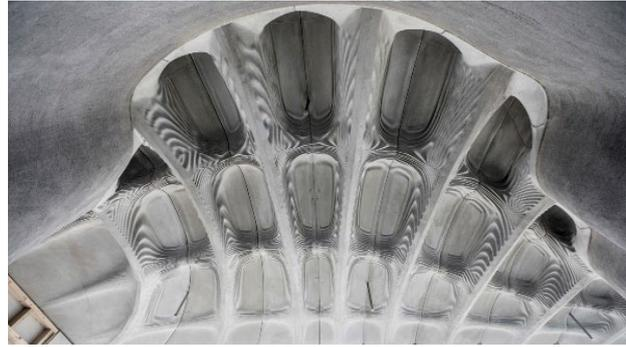
Figure 2.22 Finished Smart Slab. From (Meibodi et al., 2018).
