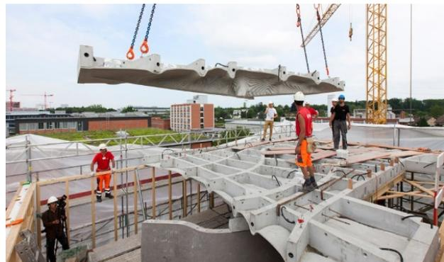
Figure 2.23 Installation of the Smart Slab. From (Meibodi et al., 2018).
