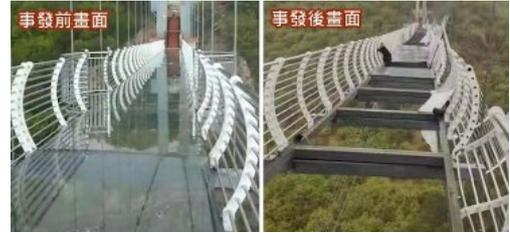
Figure 4.10 Glass bottomed bridge located in China. Before and after the collapse. From (abc.net.au, 2021).
