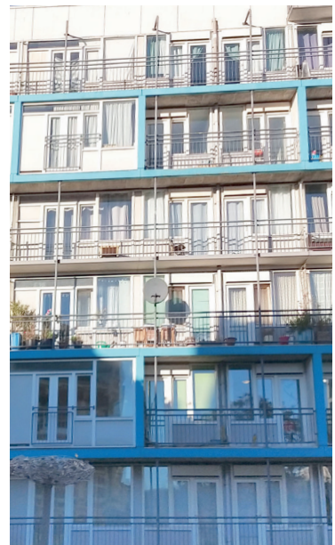
image 16. High-rise facade own photo
