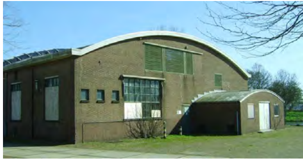
Figure 1: Low-rise Fusée Céramique vault, Woerden, The Netherlands [2].
