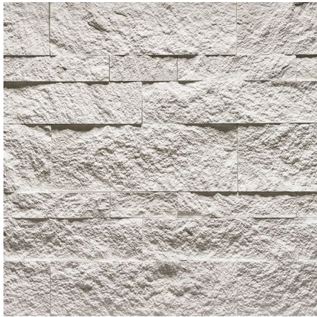
LIMESTONE MASONRY PAINTED WHITE FOR COOLING
