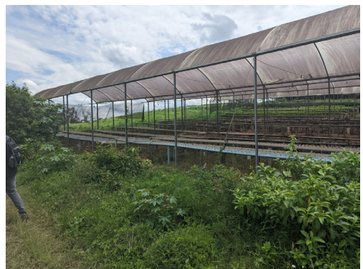
Structure for soiless agriculture with protection from excessive sun and rain
