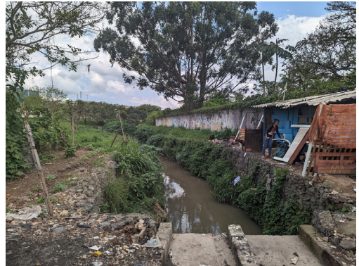
Waterbody at the end of the site parameters with informal dwelling dangerously close
