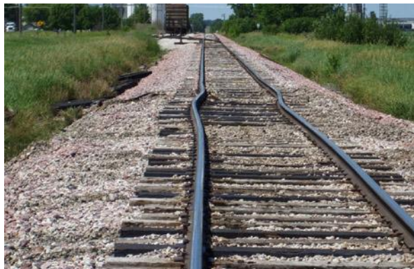
Figure 1.1: Deformed rail, (Globe Gazette, n.d.)
