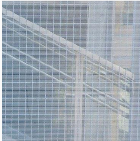
Metal mesh Facade
