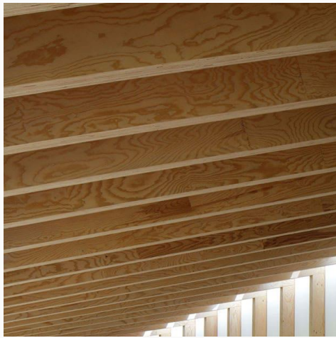
Wood Canopy / structure
