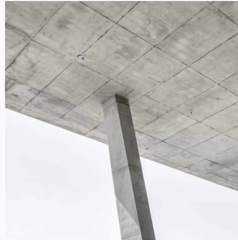
Exposed concrete Structure
