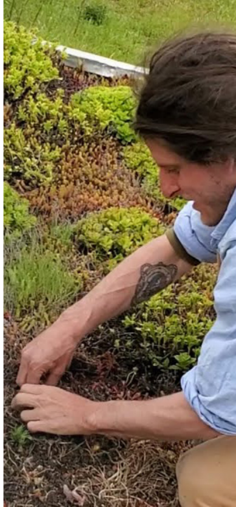
Figure 15. Weeding as part of green roof maintenance.
