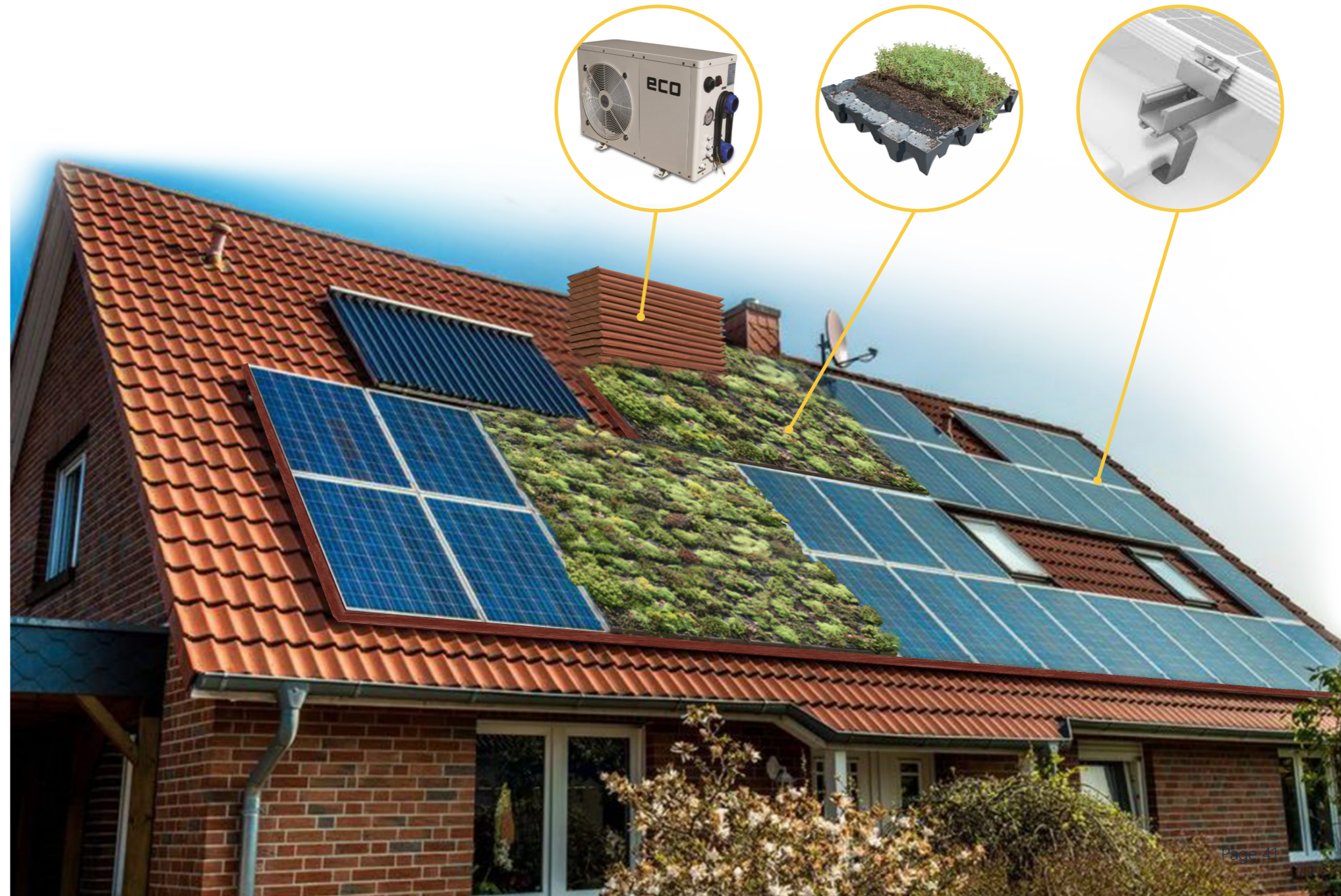
Figure 34. Concept result of cycle 2, with special attention for the heat pump, the sedum trays and standard roof anchors.
