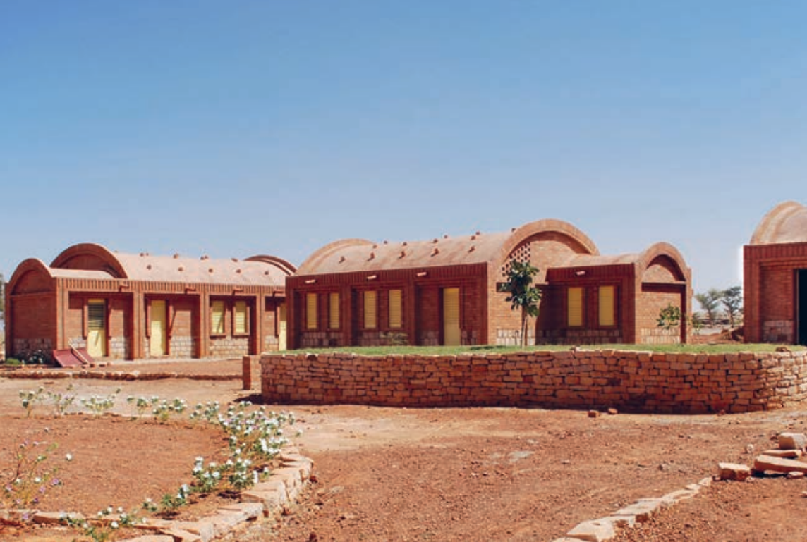
Practical Training College Sangha, Mali. LEVS Architects
