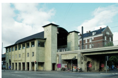
(a) Station Building from the Outside (Bloch, 2022)
