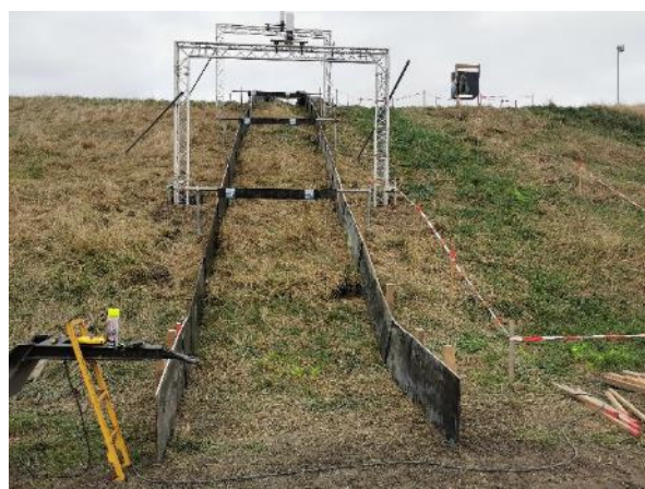
Figure 2. Standard setup of an overflow experiment, view from the landside dike toe. Camera and sensor frames are placed across the 2 m wide test section, prior to execution.
