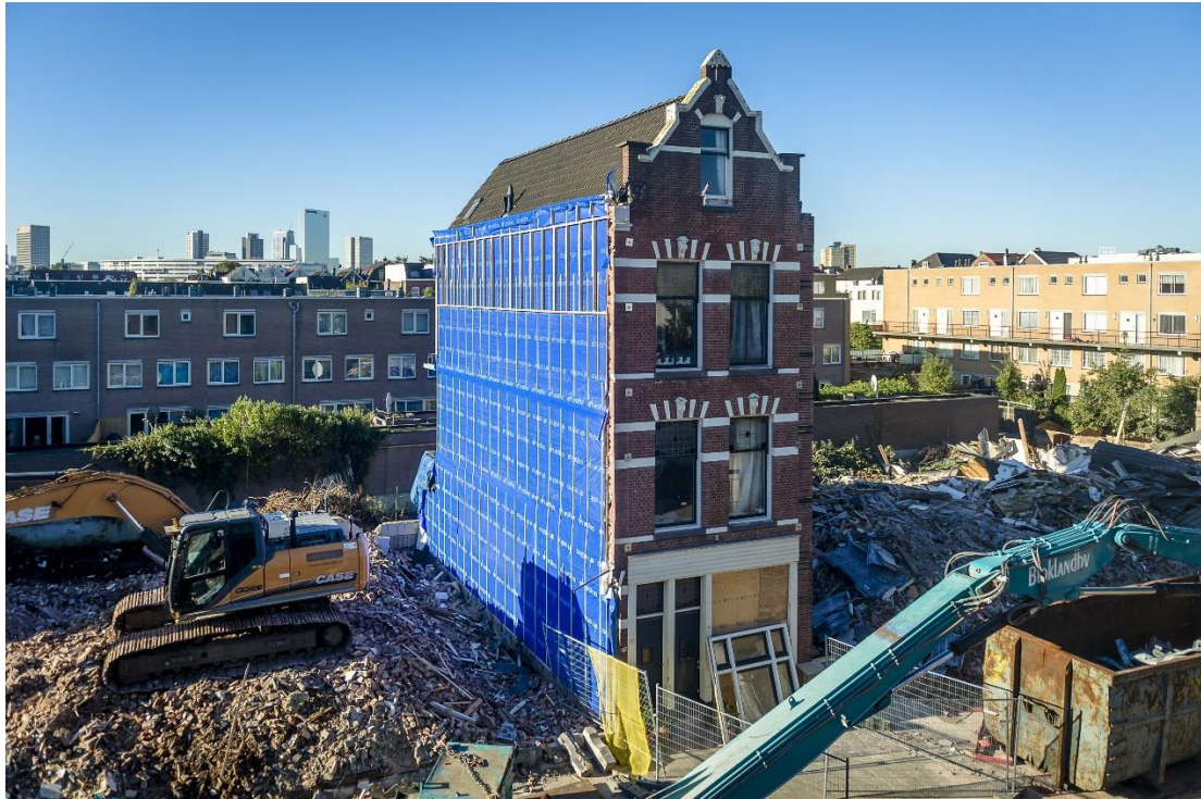
Figure 18: Combined approach of renovation and replacement, Bloklandstraat Rotterdam (Metro Nieuws, 2018)
