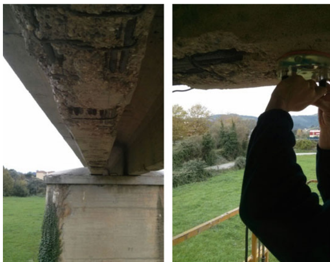
Fig. 2 Selected areas during the repair phase
