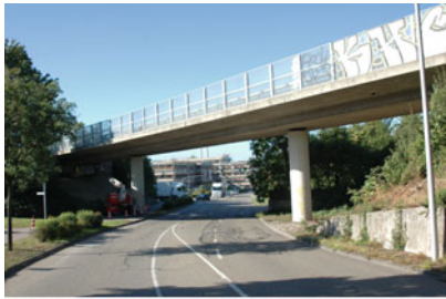
a. Overview of the bridge.
