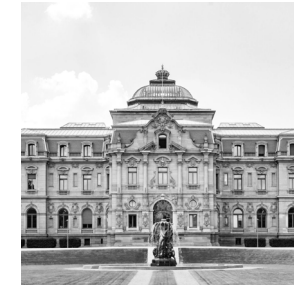
Figure 1: Federal Court of Justice Karlsruhe
