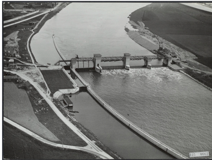
Figure 4.7: Weir-Lock complex Borgharen (KLM Aerocarto, n.d.)
