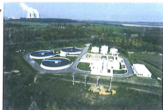
Figure 4: Mine Water treatment plant at United Schleenhain mine, MIBRAG (MIBRAG 2013).
