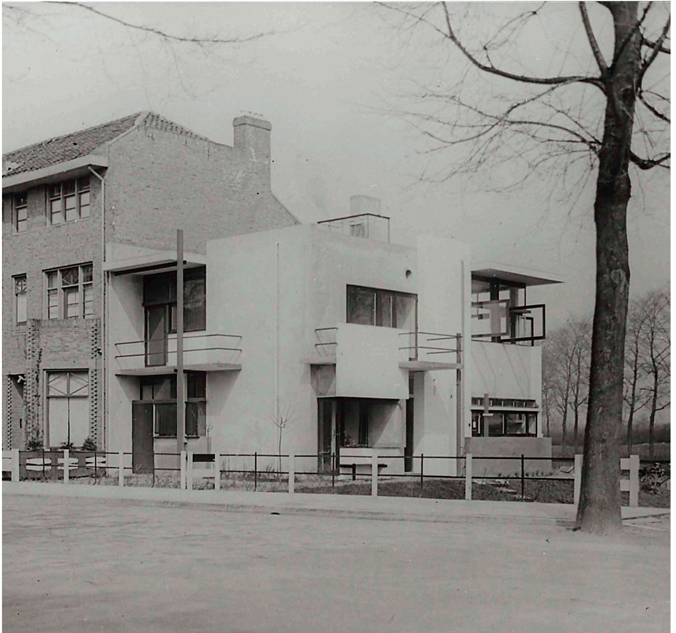
FIG. 2.1 One of the earliest photographs of the Schröder House, c. 1925
