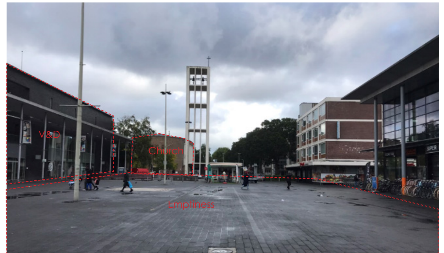
Figure 23. Photo 3 Winkelcentrum Leyweg(Bolleboom, 2023)
