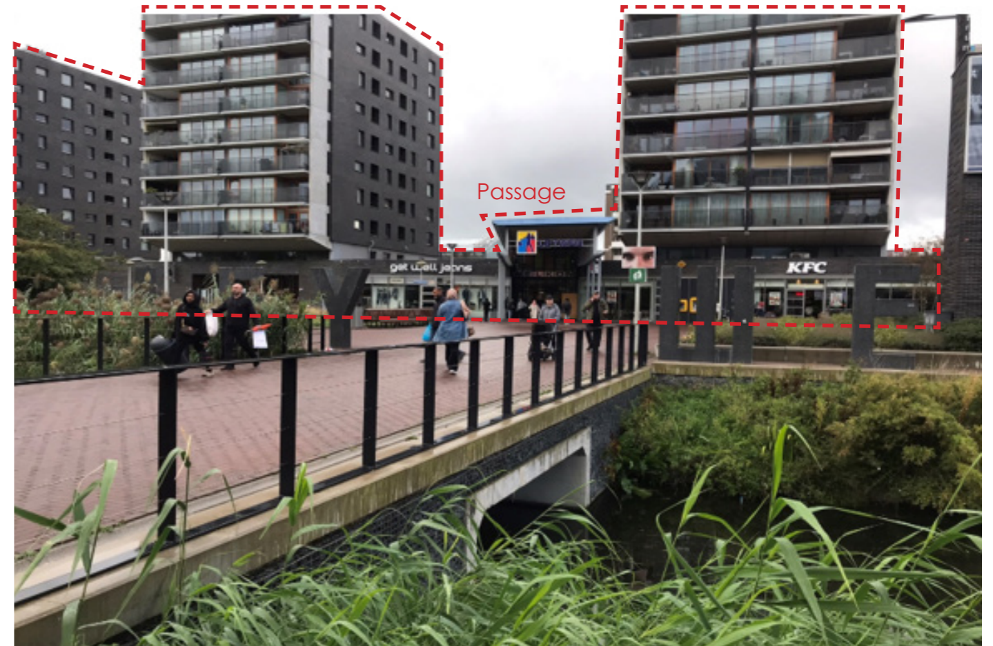
Figure 23. Photo 4 Winkelcentrum Leyweg(Bolleboom, 2023)
