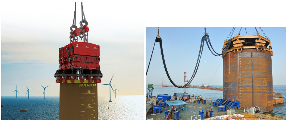
Figure 1.3: Offshore vibratory pile driving methods with large diameter monopiles
