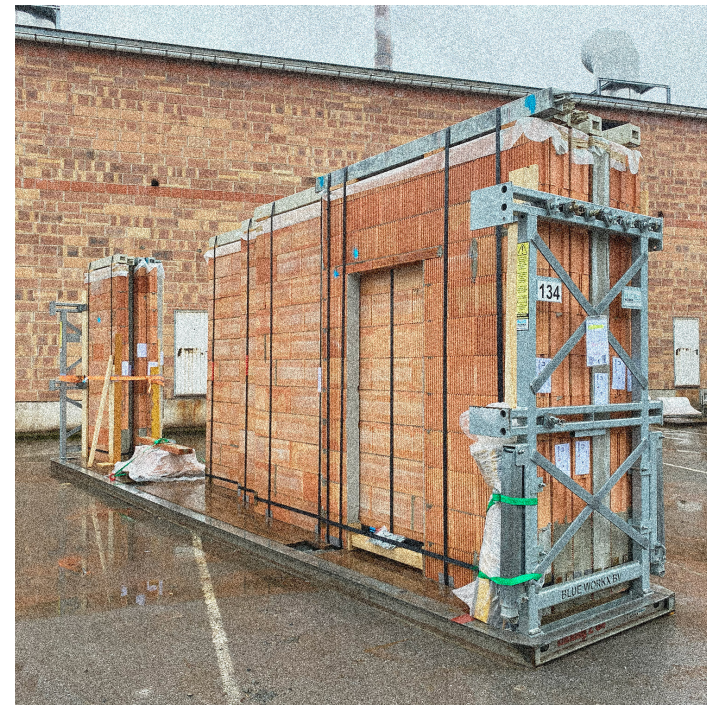
Figure 12 Multiple walls can be stored on an inloader. If stored outside, they need to be covered to stay protected from the rain.
