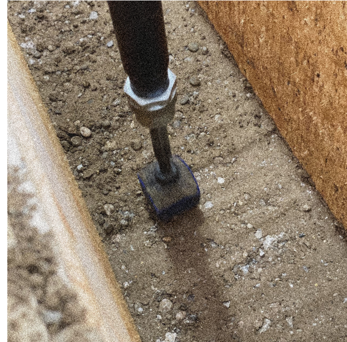
Figure 29 The robotic arm is equipped with a pneumatic rammer.
