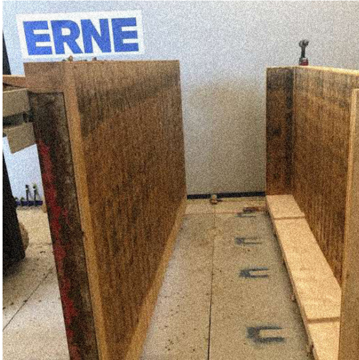
Figure 27 Formwork was conceptualized to be easily assembled and disassembled.
