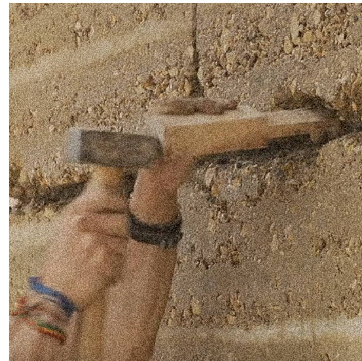
Figure 21 Once assembled using clay mortar, the joints in between elements have to be manually touched-up to be less visible and prone to erosion.
