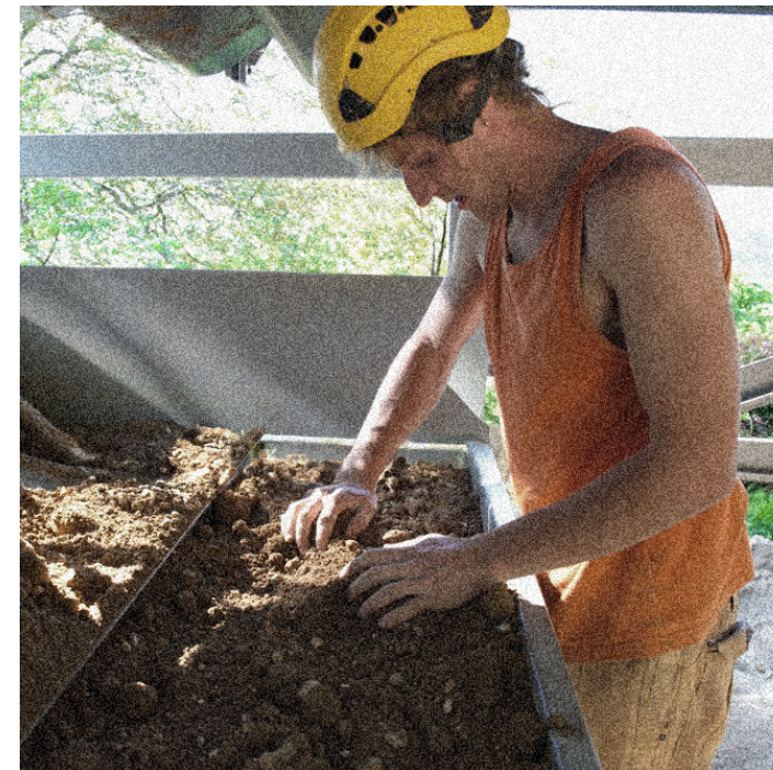
Figure 35 The final rammed earth material is portioned manually by loading a drawer, which can then be slid towards the back of the station, where the formwork is located.
