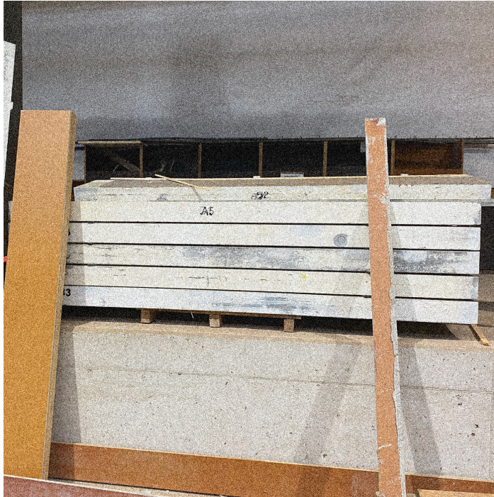
Figure 9 Formwork is applied for the elements as needed.
