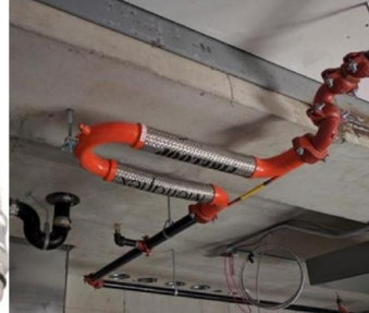
figure 2-11: Fittings for supply ducts (fvb ffc constructiv, 2000). Right: Expansion joint in sprinkler system of Brock Commons where the system exits the core (The University of British Columbia's Centre for Interative Research on Sustainability and Forestry and Innovation Management, 2017).
