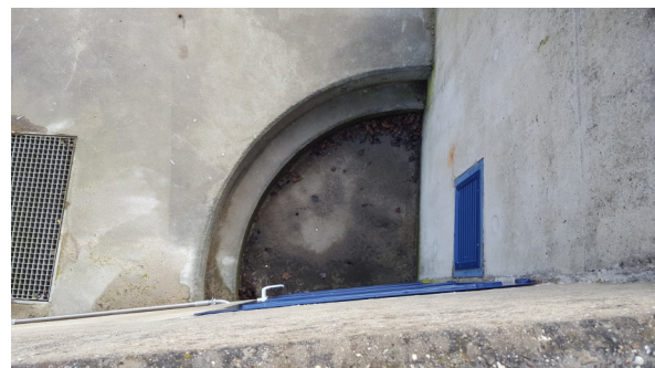
(b) Top view of maintenance entrance and part of the grating.
