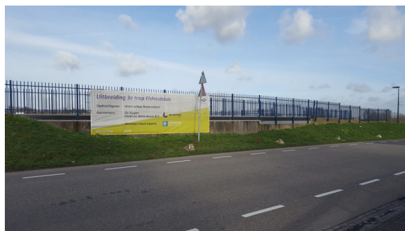
(a) The road and bicycle path on top of the Elshoutsluice with the removable bicycle path above culvert number 4.
