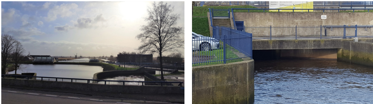
(a) The flood defences of the discharge reservoirs from the Overwaard and Nederwaard. (b) The distribution flap in the current position.
