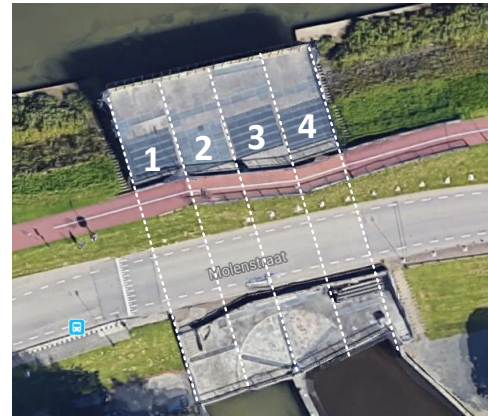
Figure 1.8: Top view of the Elshoutsluice (source: Google maps)
