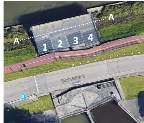
Figure 5.2: Top view of the Elshoutsluice (source: Google maps)
