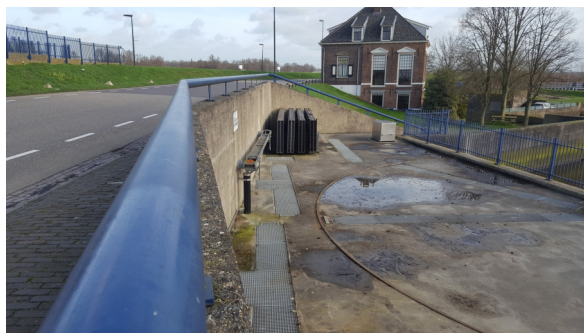
(a) The platform hinterlands of the Elshoutsluice including the grating for the weed screen.
