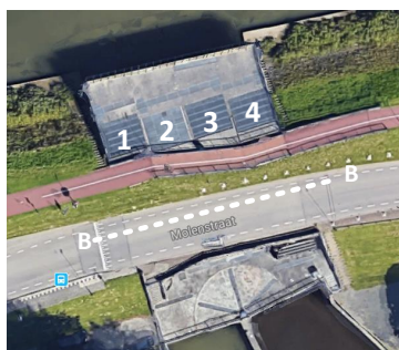
(a) Top view of the Elshoutsluice (source: Google Maps).
