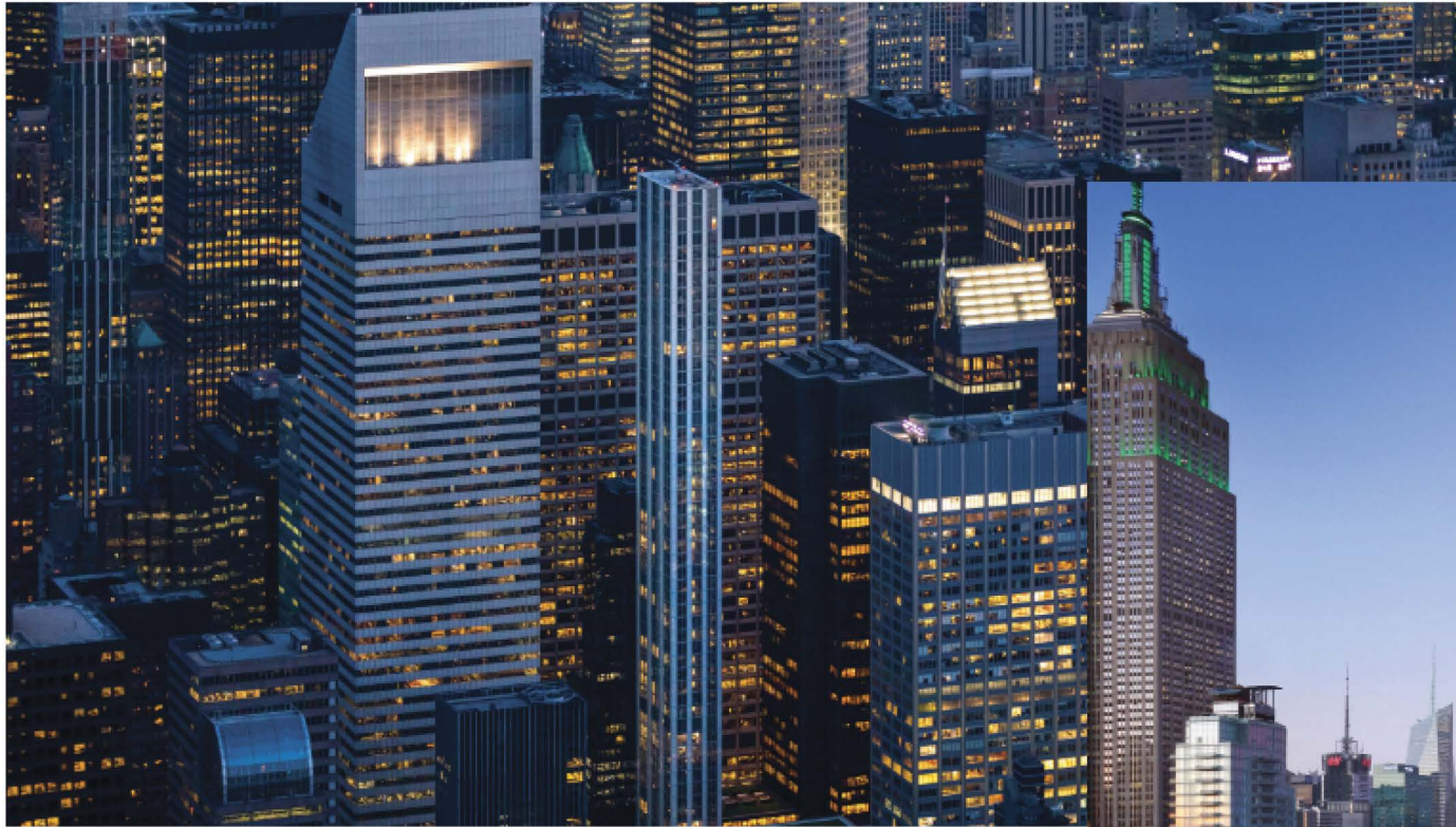
Foster + Partners' skinny New York skyscraper rises Building
