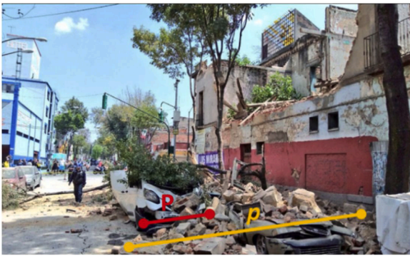
Fig. 6. Example of debris extension evaluation.
