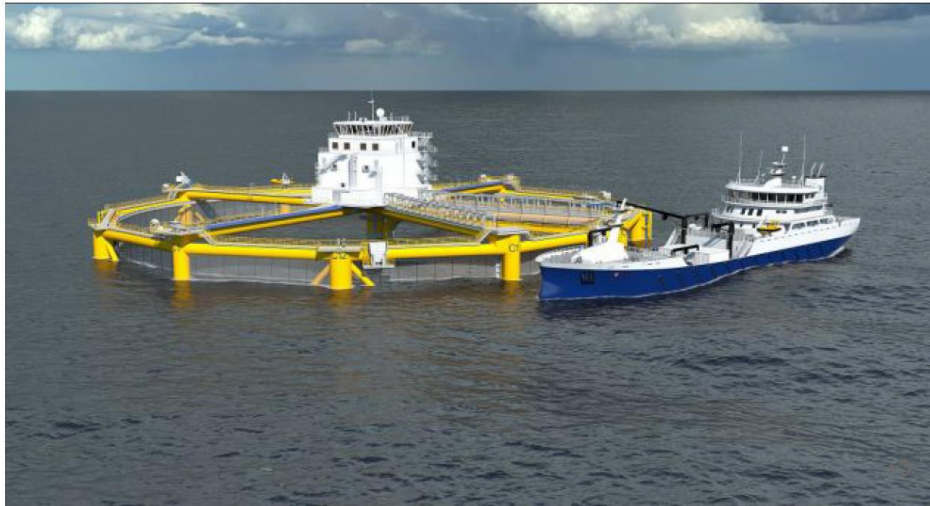
Each of the 5,600 tonne, 670-metre-high steel rigs can house eight times as many salmon as conventional cages, and the design is based on oil rigs
