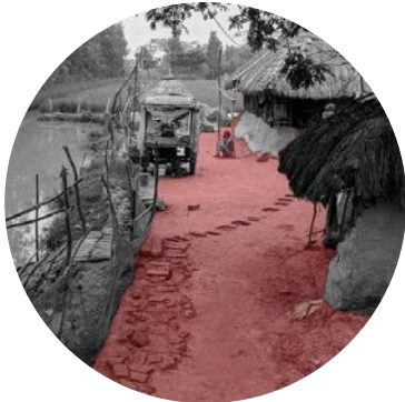
Lack of Road Infrastructure
