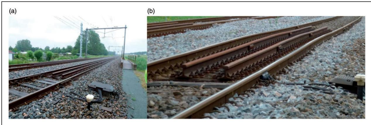
**Figure 1.** A typical track transition zone: (a) global view and (b) close-up view.
