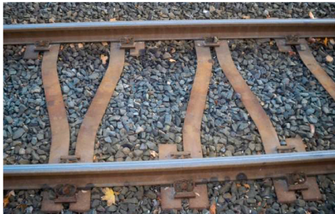
a. Y-shape sleeper (reproduced from [37])
