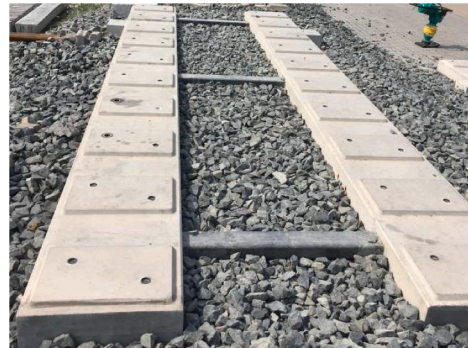
b. Ladder sleeper (reproduced from [36])
