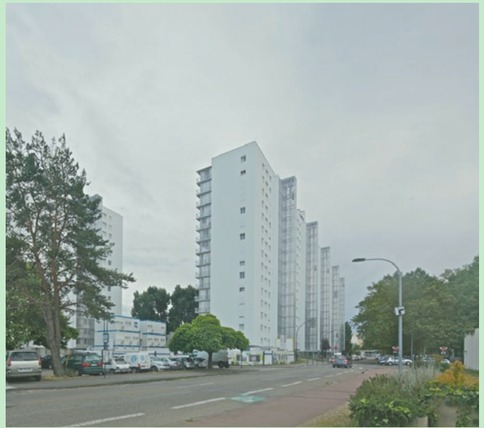
[51] New Vertical circulation on the back side. source: © Philippe Ruault
