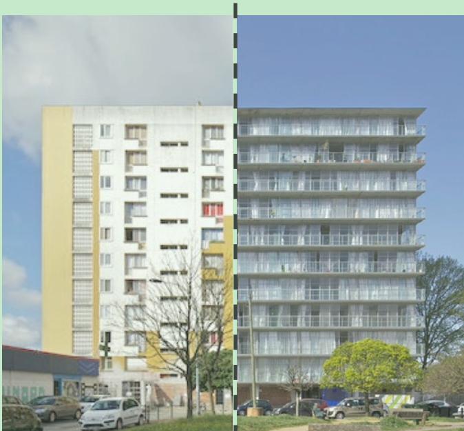
[50] Old (left) v.s. new facade (right) (the smaller building slab) source: © Philippe Ruault
