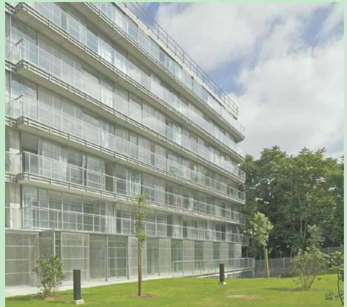
[61] Garden in the inner courtyard source: © Philippe Ruault
