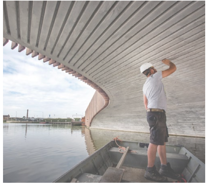
[66] cavities on the bottom side of the bat bridge source: NEXT Architects
