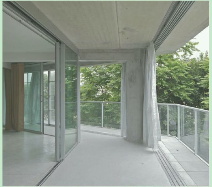
[64] Wintergarden as an extension source: © Philippe Ruault
