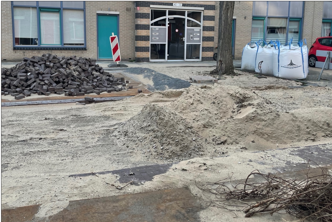
Understanding the infrastructure of a street in Delft (February 2023)
