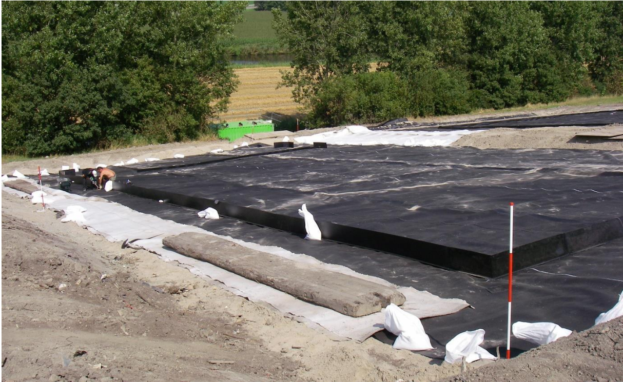
Figure 30: Bottom and side walls of test field
