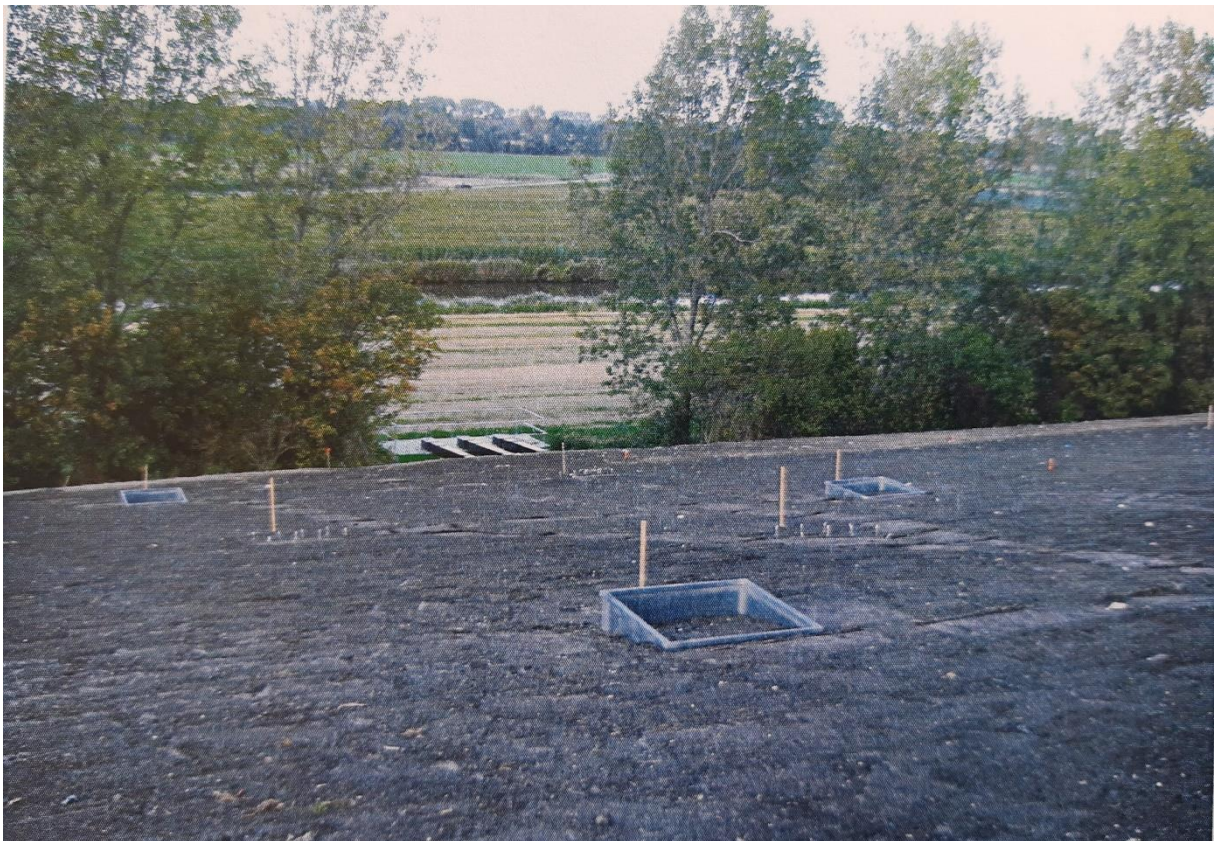
Figure 35: View at end of construction. The boxes and tubes emerging from the field were used by the landfill gas experiments.
