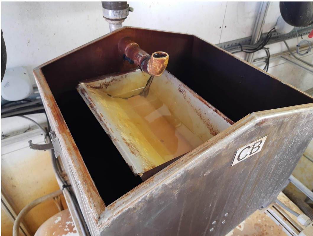
Figure 43: The tipping bucket of the capillary block.
