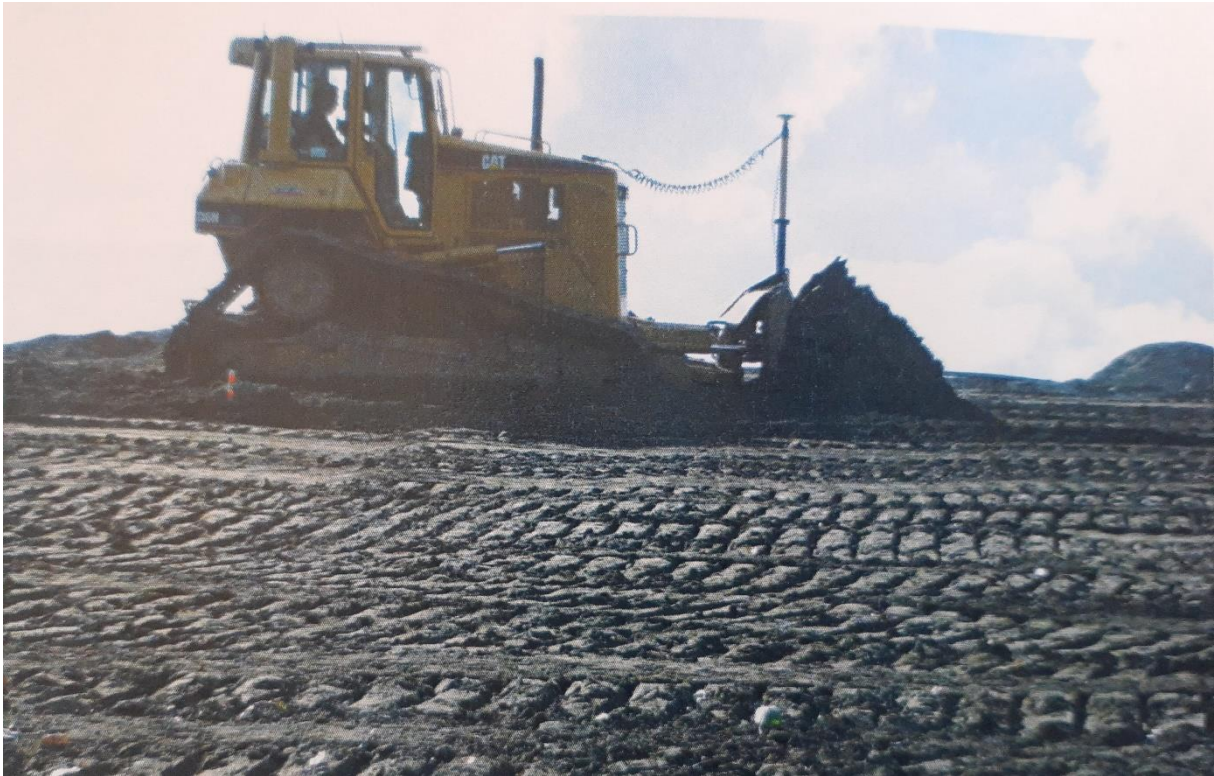
Figure 36: Construction of top 60 cm of the MOL with a bulldozer.
