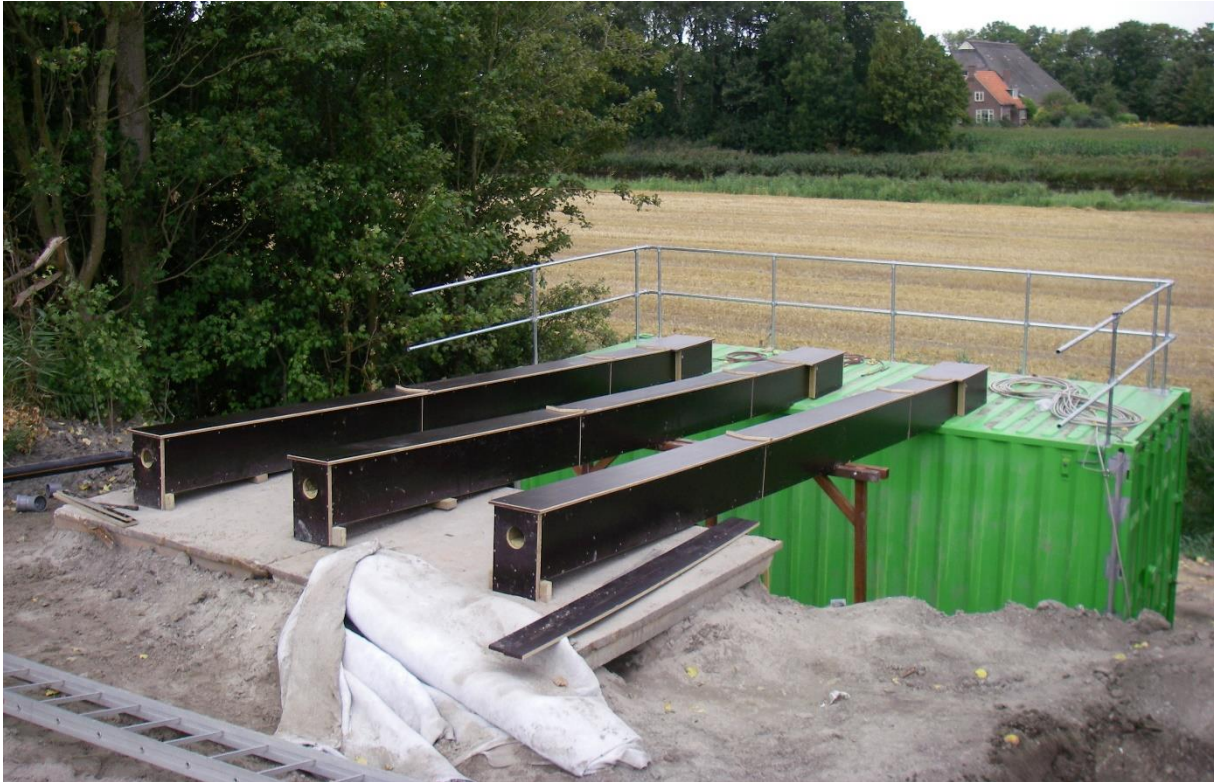
Figure 32: Bridge for drains to the measurement container
