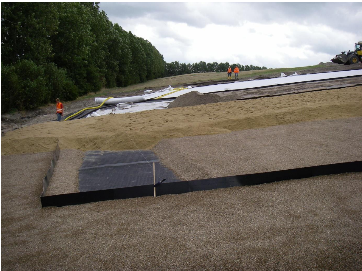
Figure 33: Construction of the capillary layer.
