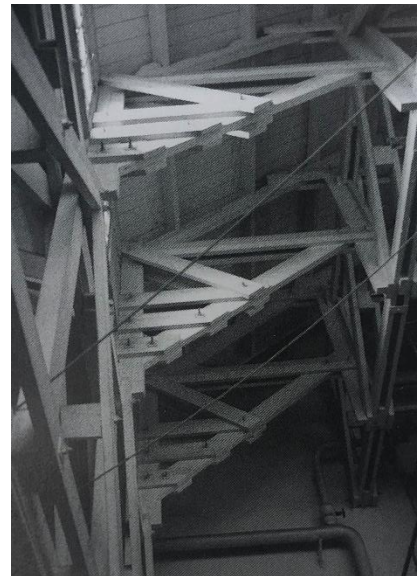
Figure 3.4.1 – Picture beams Decontamination building (Moscoviter, 1993)
