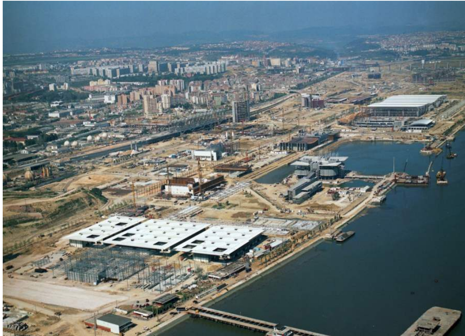
Expo '98 pavilion - during construction
