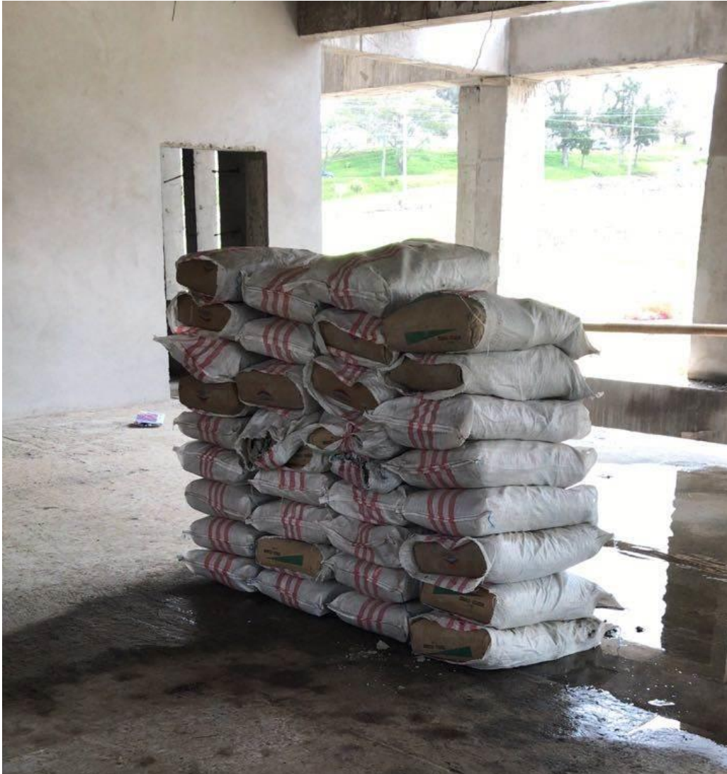
Figure 13. Example of application of dead weight with cement bags. Photograph by S. Camino. Printed with permission.
