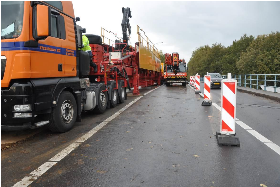
Figure 3. Proof load test on viaduct where one lane of traffic (right side of photograph) remains open for traffic (Fennis et al. 2014, Koekkoek et al. 2015).
