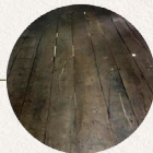
Wooden Floor (Reused from Shutte boards and column boards)
